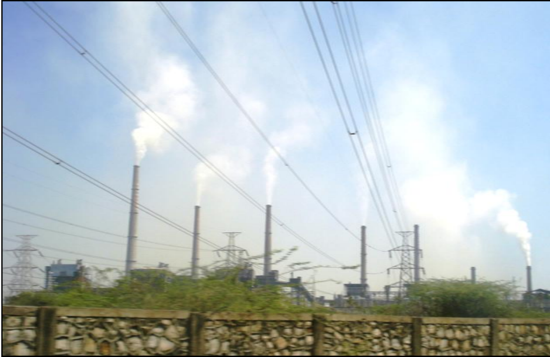
Photo 1: Stack Emissions from 2340 MW Chandrapur Super Thermal Power Station (Mahagenco)
